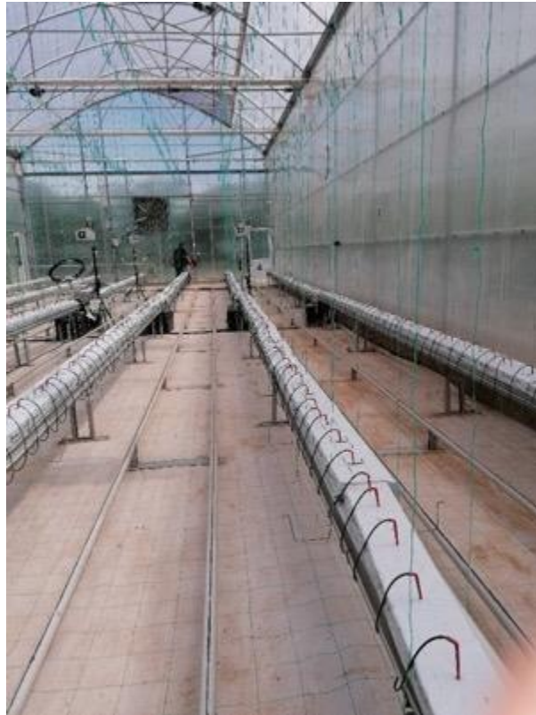
Figure 6. Heat distribution system
